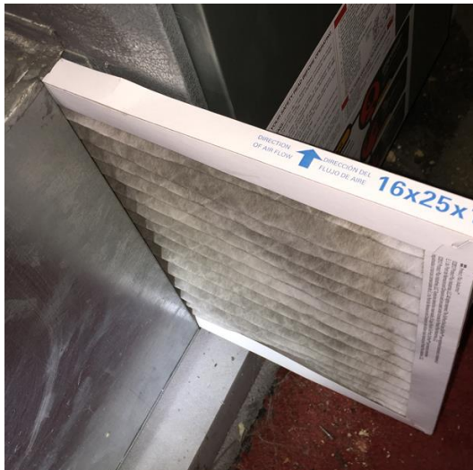
Air filters replacement
